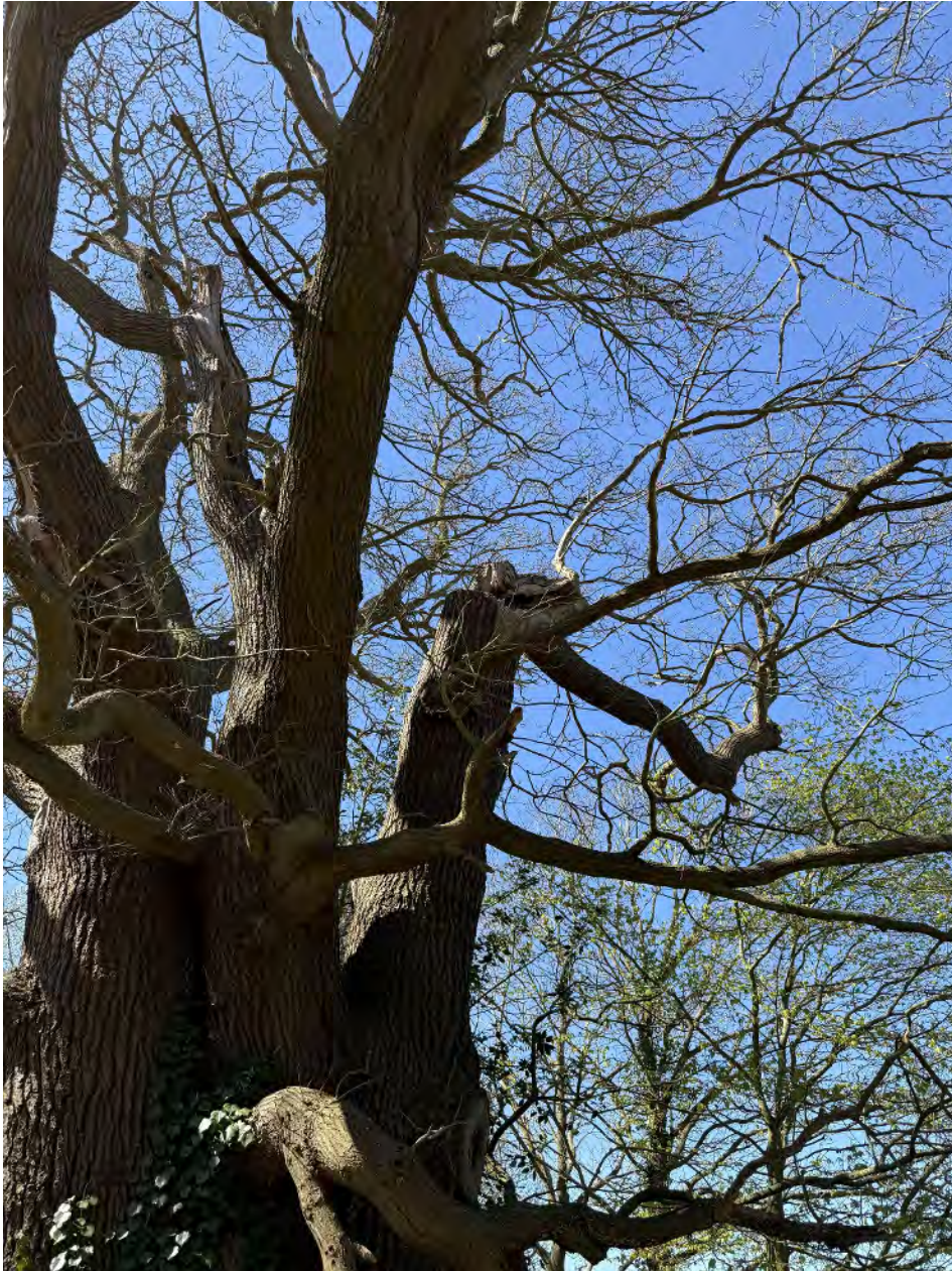
Image 3 - T30 Decayed scaffold structure
